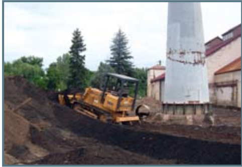
Cleanup underway at the Durango Powerhouse in Durango, Colorado
