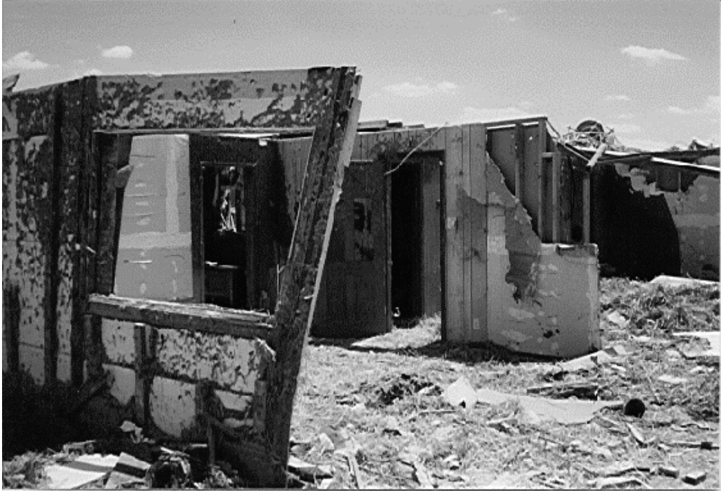
Remains of a home adjacent to the Double Creek Estates subdivision of Jarrell. This home is located on the edge of the tornado path. Five people survived the storm in a bathroom (center of picture). Photograph by E. L. McIntyre, NOAA/NWS.
