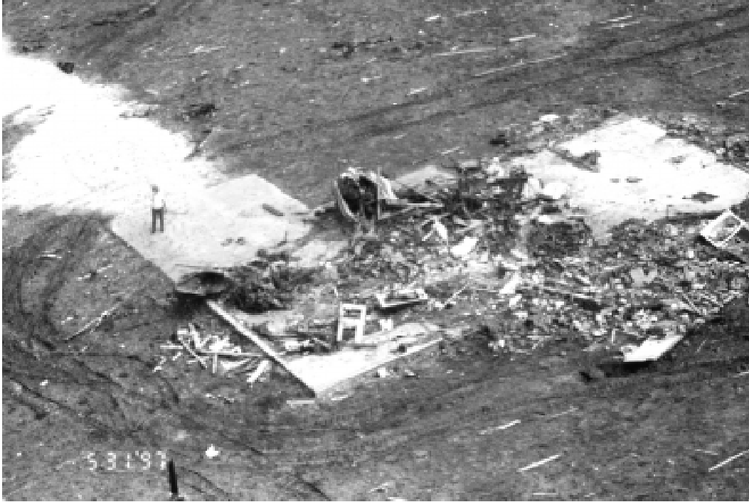
Close-up aerial view of the remains of a home in the Double Creek Estates subdivision of Jarrell. Photograph by L. Phan, NIST.
