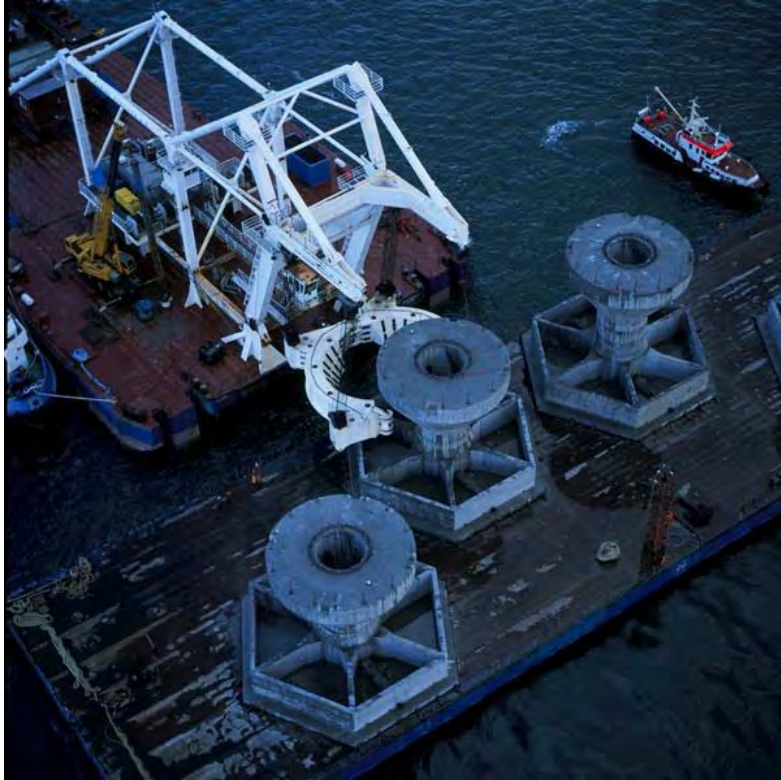
Figure 2.8. The Eide Barge 5 Lifting a Gravity Foundation at Nysted
