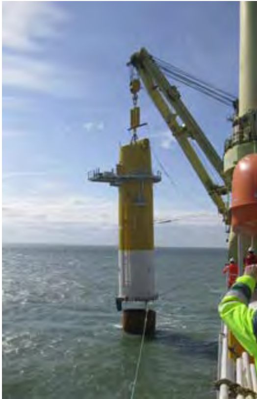
Figure 5.4. Transition Piece Being Placed over Monopile
