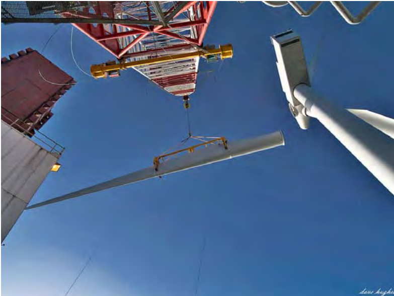
Figure 5.8. Installation of a Single Blade at Lynn and Inner Dowsing
