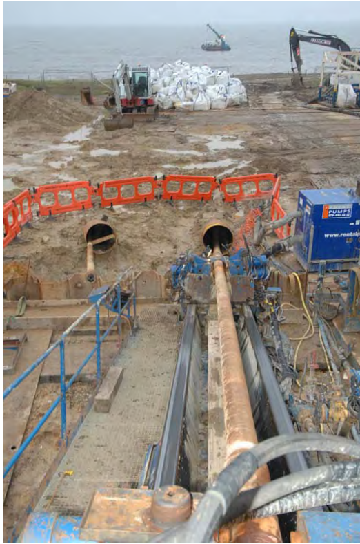
Figure 5.16. Horizontal Directional Drilling at Sheringham Shoal
