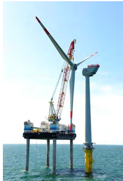
Figure 5.10. Installation of an Assembled Rotor at Alpha Ventus Source: Alpha Ventus 2010
