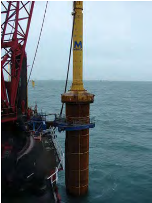
Figure 5.2. Hammer Placed on the Top of a Monopile Before Driving
