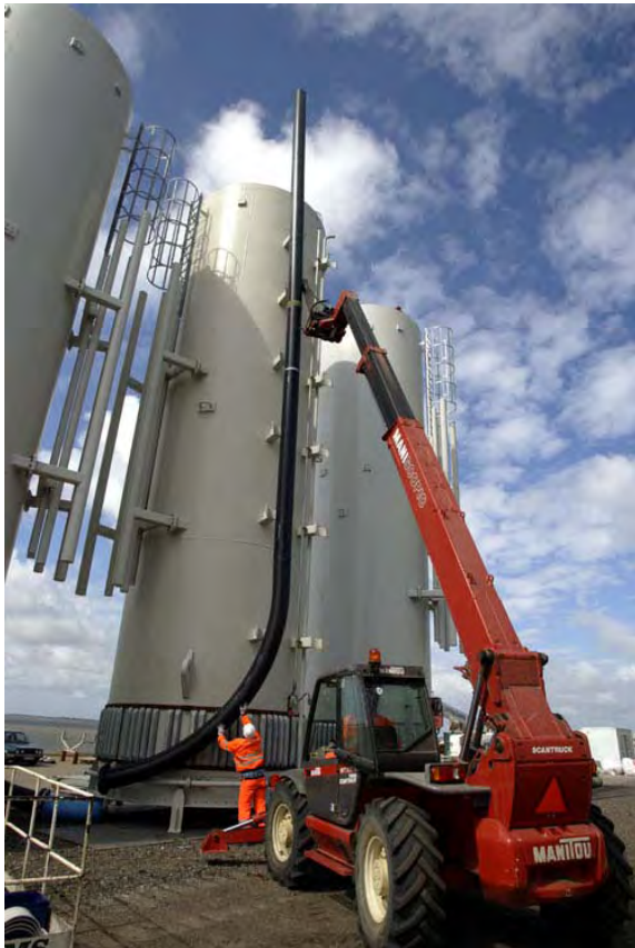
Figure 5.15. A J-Tube Being Installed on a Transition Piece
