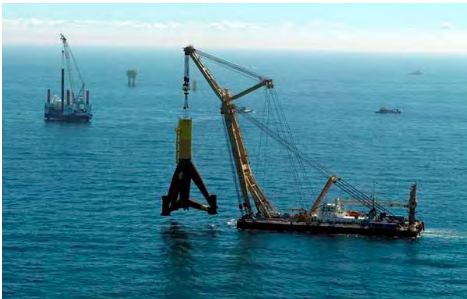
Figure 5.5. The Taklift 4 Placing a Tripod Foundation at Alpha Ventus
