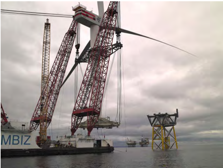
Figure 5.13. The Rambiz Installing a Fully Assembled Turbine at Beatrice
