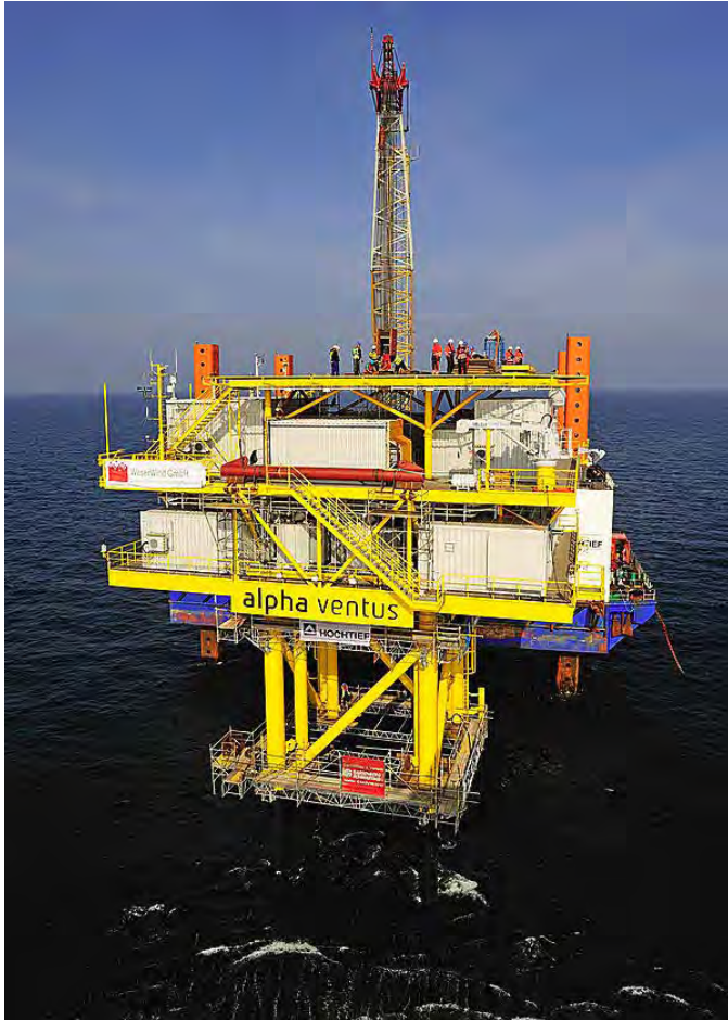
Figure 2.6. A Jacket Structure Supports the Substation at Alpha Ventus
