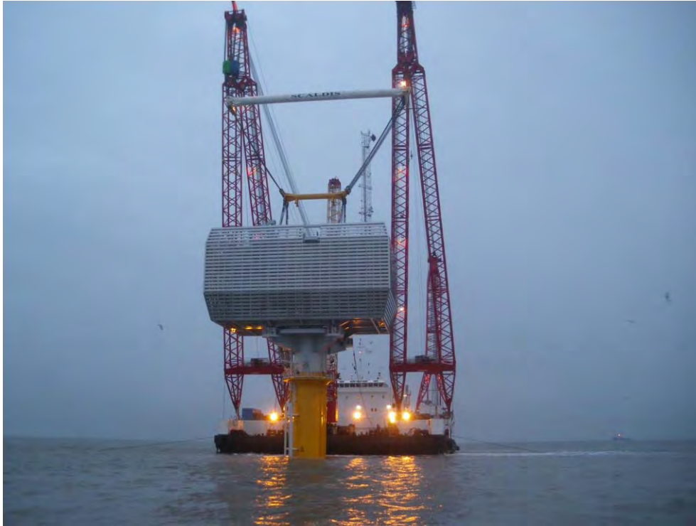
Figure 2.17. Substation Being Lifted onto Monopile at Gunfleet Sands
