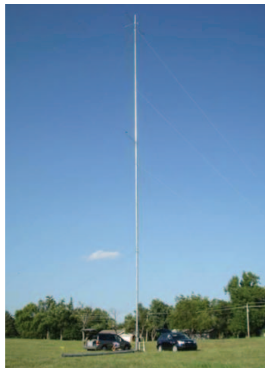
In preparation for installations at chosen sites, John Brown University staff temporarily installed a meteorological tower on the campus to check and calibrate the equipment. Photo credit: Jenny Ahlen.
