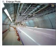
Photo courtesy of Brookhaven National Laboratory Brookhaven National Laboratory's Relativistic Heavy Ion Collider (RHIC) is really two accelerators in one—made of crisscrossing rings of superconducting magnets, enclosed in a tunnel 2.4 miles in circumference. In the two rings, beams of heavy ions are accelerated to nearly the speed of light in opposite directions, held in their orbits by powerful magnetic fields.
