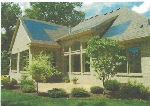
Although a south-facing orientation is best, solar systems will perform well at different orientations, as this Ohio home demonstrates.
