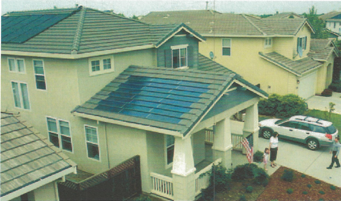
This solar home in Davis, California, uses EnergyTiles ® made by BP Solar.
