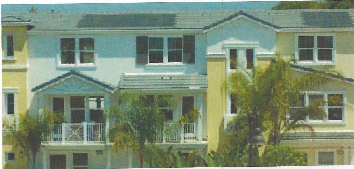
A 1-kilowatt solar electric system was integrated into the roof of each of the 77 units in this housing development in San Diego, California.
