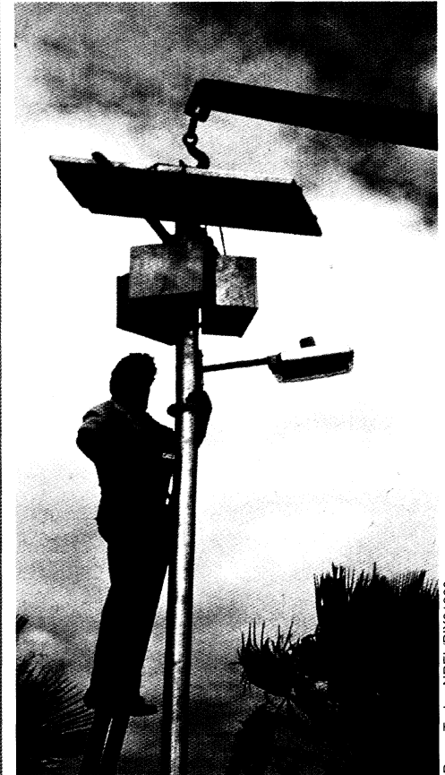
Worker installing a grid-independent, PV-powered street light.
