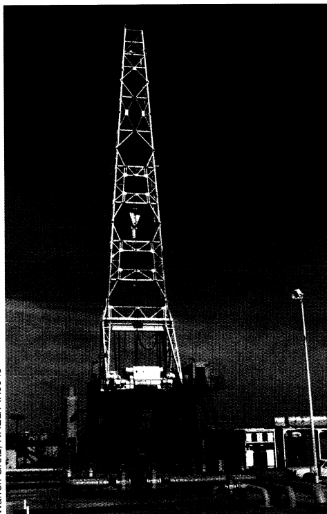
Geothermal production well at Imperial Valley, California.
