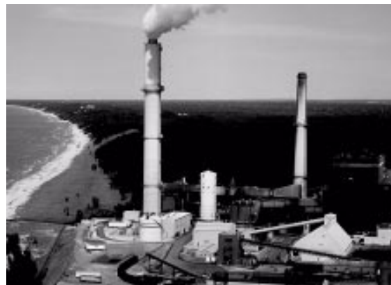
Equipped with the Pure Air advanced desulfurization unit, the Bailly Station on the shores of Lake Michigan is now removing more than 95 percent of the sulfur pollutants from its coal combustion flue gas.
