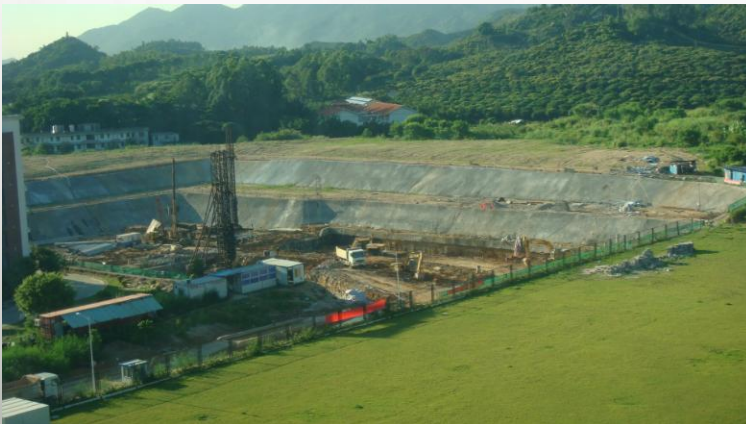
Nebulae's New Home – National Supercomputing Center in Shenzhen, China
