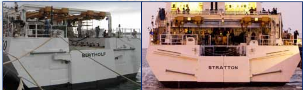
The Bertholf’s original stern doors, left, were modified to match the Stratton’s stern door configuration, right. U.S. Coast Guard photos.
