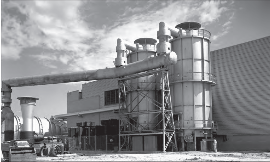
Image 56: Depending on the type of test being run, the airflow into the engine would have to be either heated or refrigerated. Ramjets operated at supersonic speeds and needed to be tested in hot conditions to simulate the heat generated by their velocity. Ambient air was taken into these two heaters and passed through natural-gas-heated vertical tubes. Each heater warmed 125 pounds of air per second degree Fahrenheit. 11 (NASA C-1952-30936)
