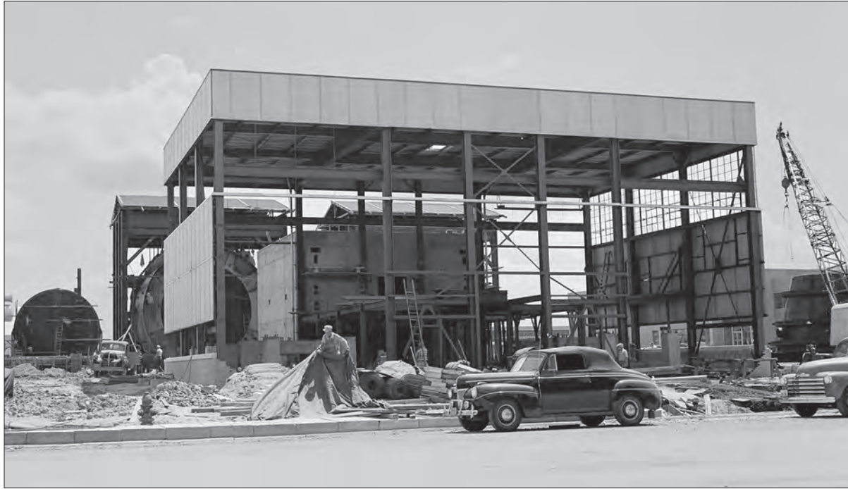
Image 24: Early stages of construction of the Shop and Access Building in August 1950. The two altitude chambers and control room would be added to the second floor later. (NASA C-2009-00179)
