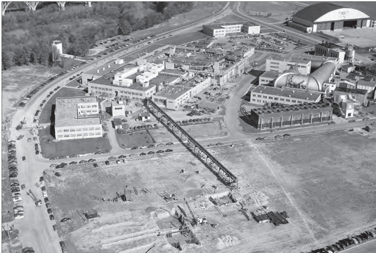
Image 20: Future site of the PSL as it appeared in October 1949. A process air line is seen being built from the Engine Research Building to the PSL site. The AWT is near the upper right corner of this photograph. (NASA C-1949-24972)
