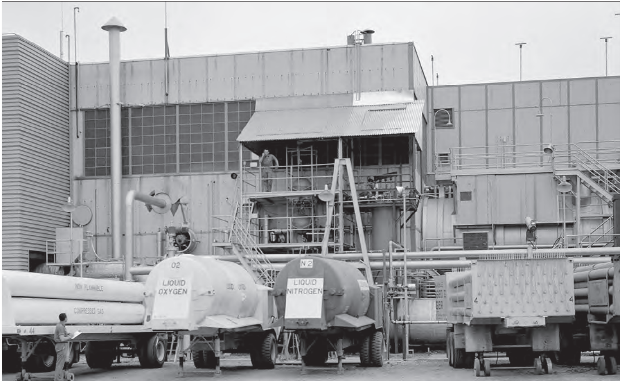
Image 106: Liquid-oxygen and liquid-hydrogen tanks brought in for a PSL rocket test on 16 April 1963. The control room is inside the building to the right of the awning. (NASA C-1963-64268)
