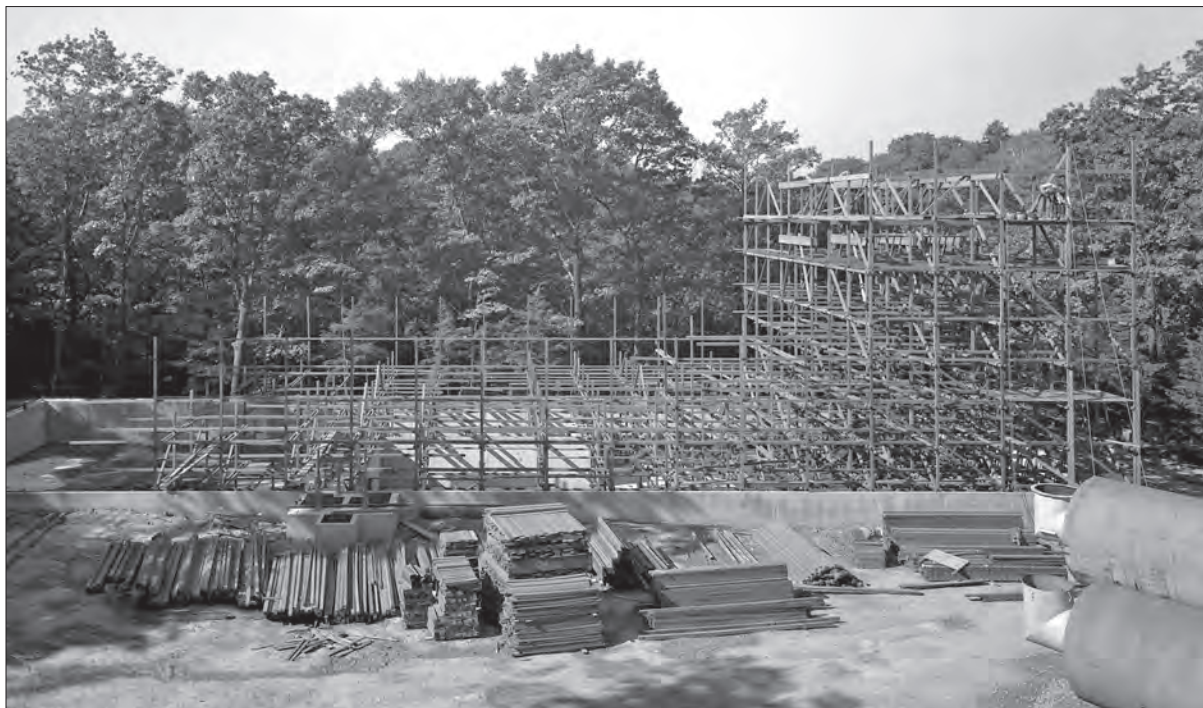
Image 32: Construction of the wooden PSL Cooling Tower in a wooded area across the road from the PSL in September 1949. (NASA C-2009-00161)
