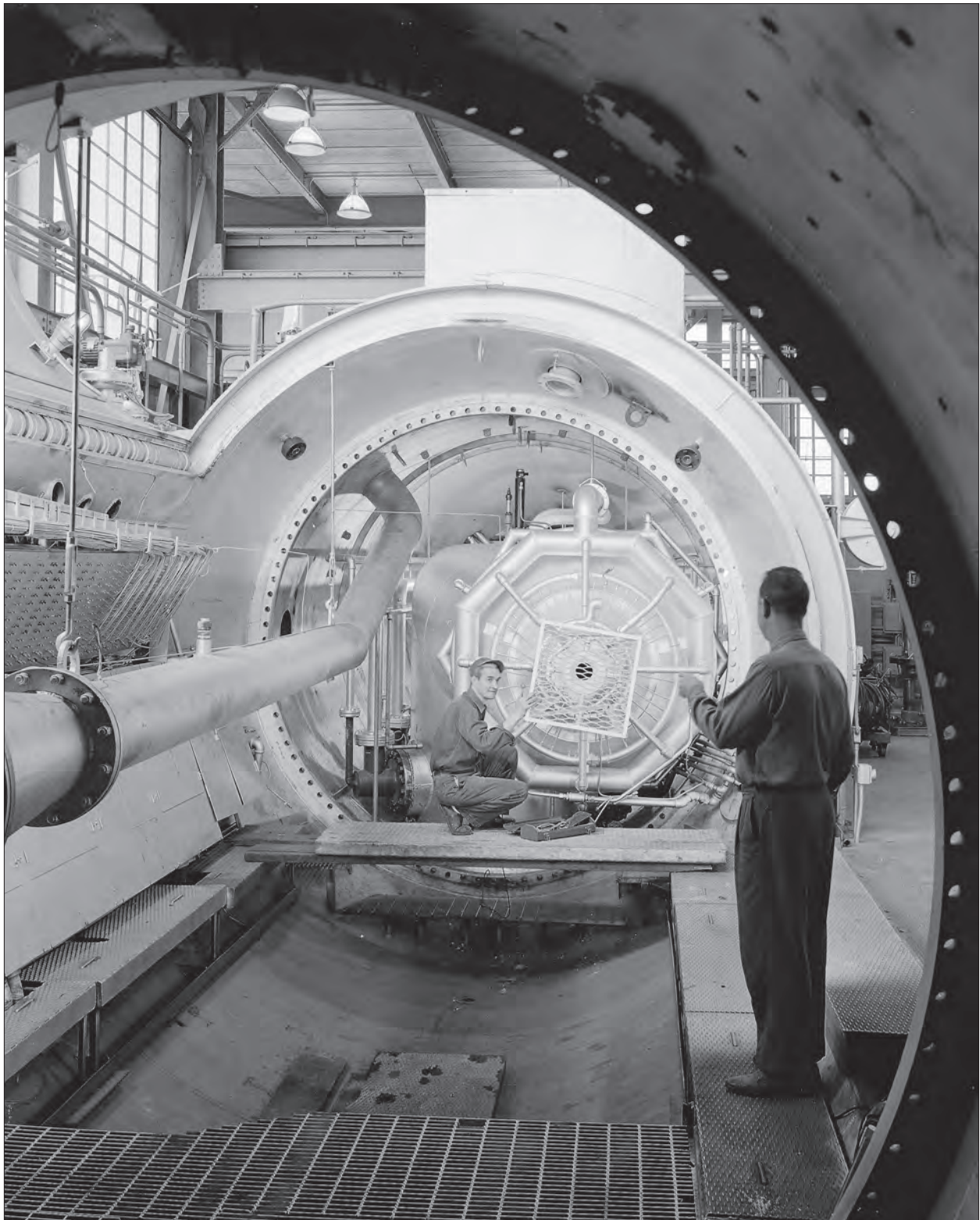
Image 95: Work on the pebble bed heater's inlet nozzle on 15 November 1958. The heater was active in May, and the tunnel was operational in July. (NASA C-1958-49138)
