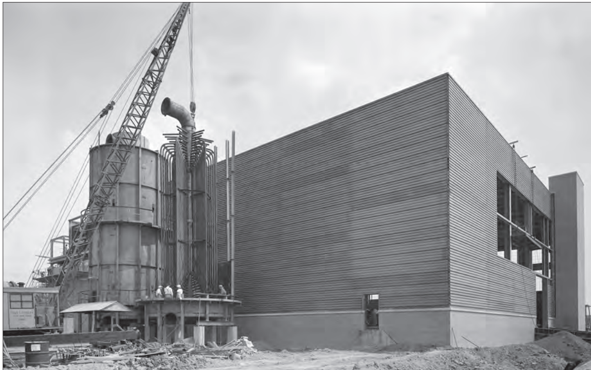
Image 31: Construction of the gas-fired air heaters outside the Equipment Building on 29 August 1951. (NASA C-2009-00163)
