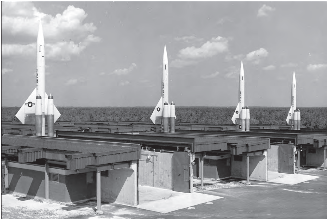
Image 83: Squadron of Bomarc missiles in the 1960s, each with its two 24-inch-diameter Marquardt ramjets visible. Ten missile sites with a total of 500 weapons were deployed around the perimeter of the United States, including two Canadian sites. (U.S. Air Force)
