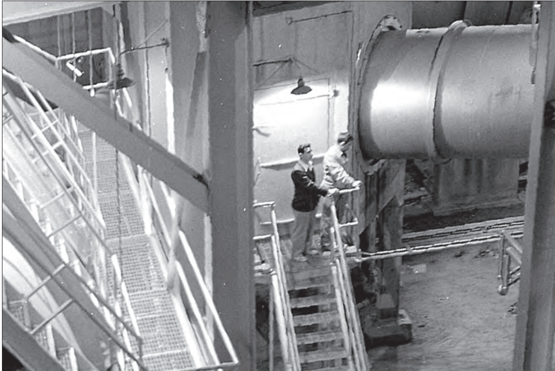
Image 50: The third shift would come in overnight to actually run the tests. The facility required so much electricity that the NACA had an agreement with the local electric company to operate the facility only at night. Many of the researchers did not care for the late-night testing and sought out operational engineers to run the tests. (NASA C-1952-30766)
