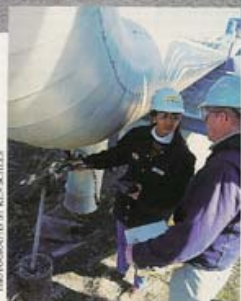
JUST BY CHECKING steam traps like the one at left, Du Pont saved $1 million a year at its vast Chambers Works (above) in New Jersey.
