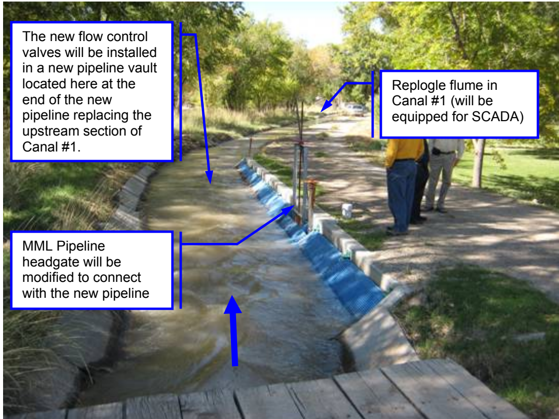
Figure 13. Canal #1 at the entrance to the MML Pipeline (looking downstream). A new concrete vault with flow control valves will be installed at the junction with the MML Pipeline.
