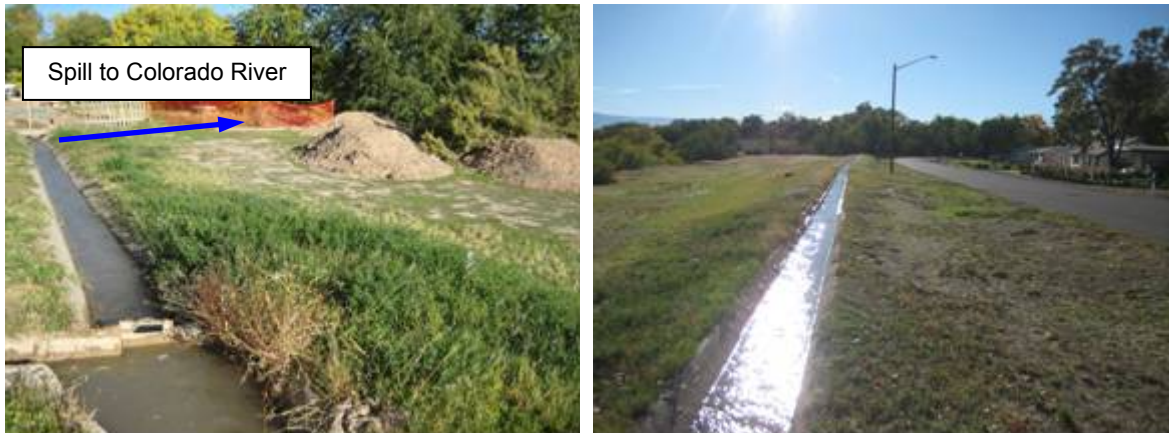
Figure 25. End of the MML system. The MML spills to the Colorado River at the site shown on the left.
