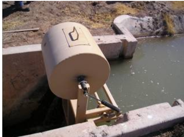
Figure 22. ITRC Flap Gate installed in a canal spill structure (Imperial Irrigation District, Calif.)
