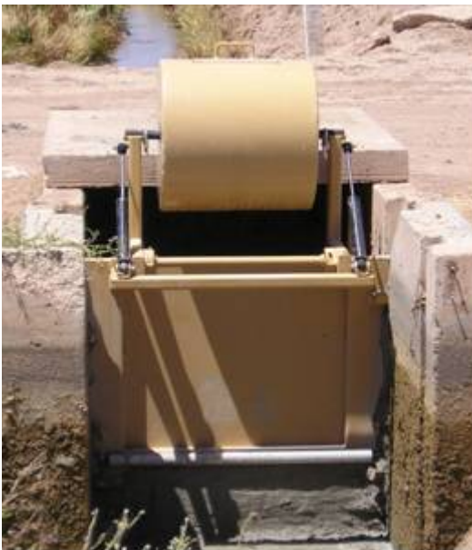
Figure 22. ITRC Flap Gate installed in a canal spill structure (Imperial Irrigation District, Calif.)
