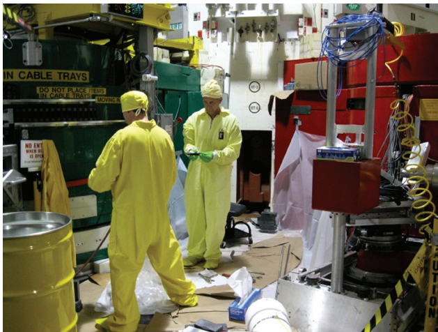
Paul Liposky and Jim Moody work on the RT-4 pneumatic transfer system.
