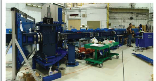
➤ The new guides are pre-aligned and assembled in the high bay to expedite installation in C100.
