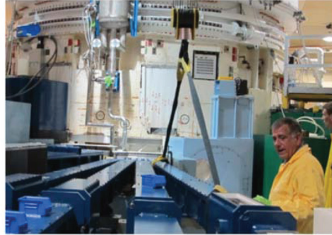
▲ Mike Rinehart and Doug Ogg (l-r) re-install the NG-1 vacuum jacket in C-100. The first guide elements of existing guides NG-1 thru 7 were replaced as part of the refurbishment program.
