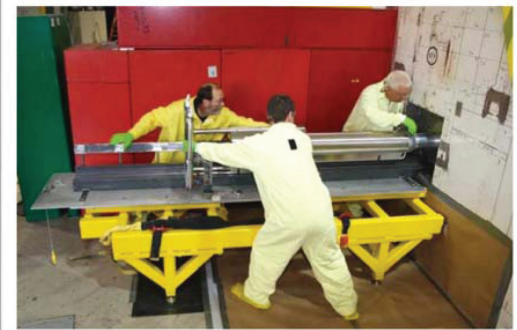
▼ ...during installation of the new cold source.
