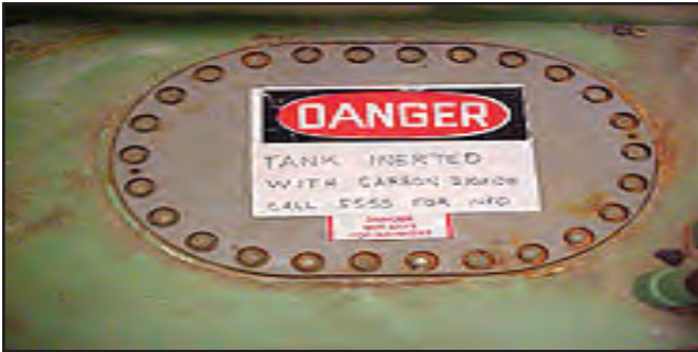
Photograph of proper signage used to indicate the designation of an enclosed or confined space.
