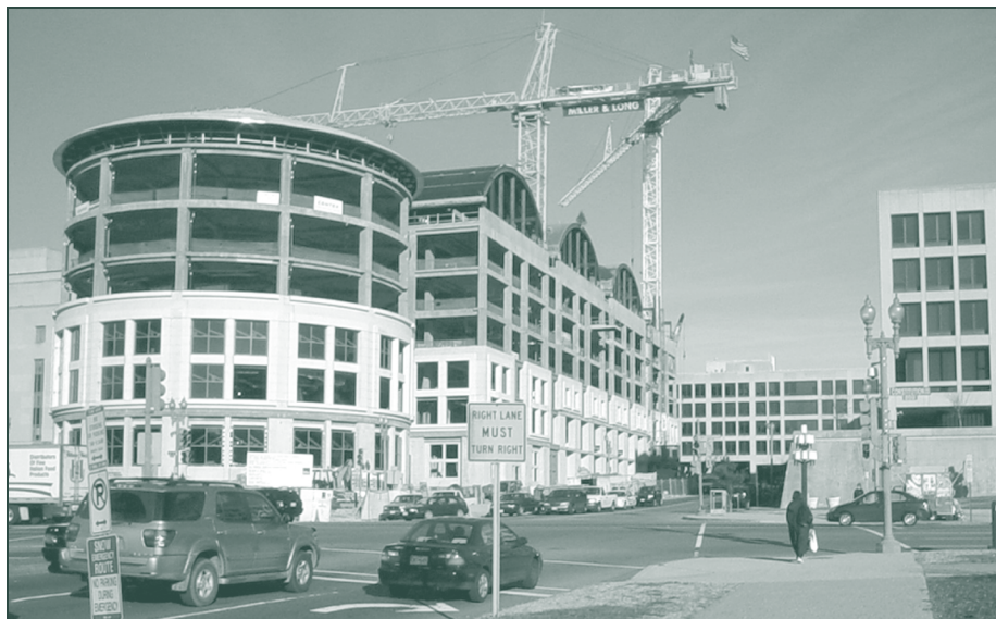
Construction of the E. Barrett Prettyman U.S. Courthouse Annex is underway.
