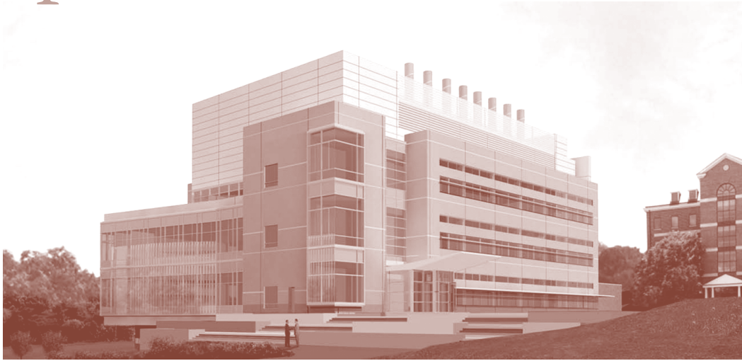
A new laboratory building at the National Institutes of Health will be clad with a variety of materials, including brick, glass, and metal panels.
