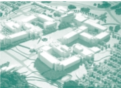
Two projects included in the FCIP are the National Institutes of Health's clinical research center (left) and the Food and Drug Administration's White Oak consolidation (above), both in Montgomery County, MD.
