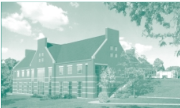
The new fire station at NIH in Bethesda
