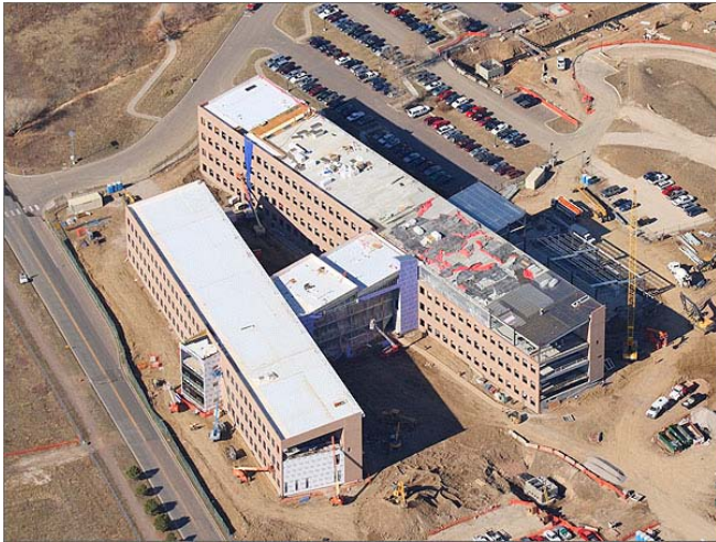
Figure 4 The “lazy H” configuration of two narrow multistory office wings (connected by an enclosed bridge and courtyards) allows daylight to penetrate the work spaces.
