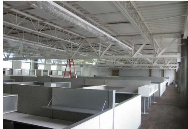
Figure 5: RSF Construction Photo
