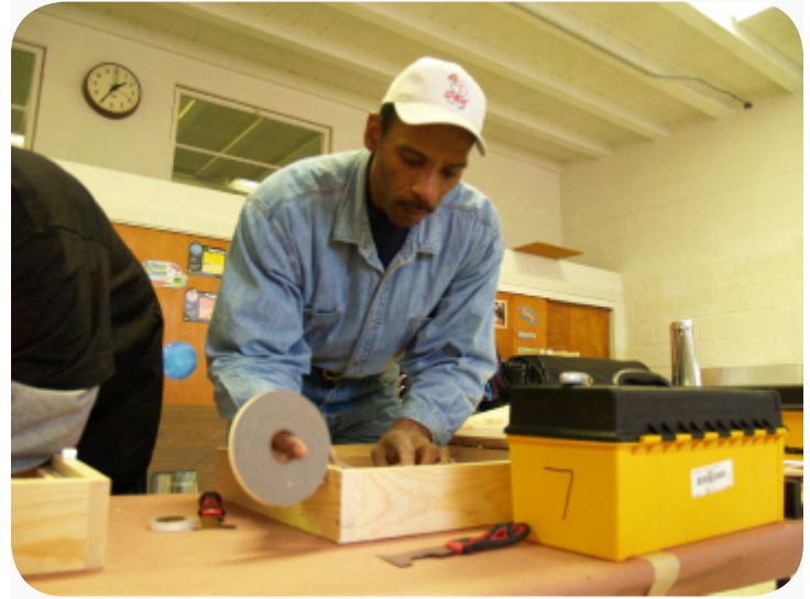
Kelvin Reaves air sealing attic hatch.
