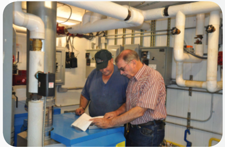
Billy Lowery (left), HVAC installer at Davis Godwin Associates, Inc.
