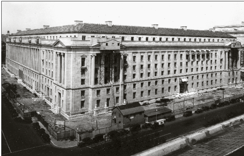
Construction photograph taken August 1934, showing the 10th Street and Constitution Avenue fronts of the building. Note the platform along the parapet on the 10th Street side and the pediments on the Constitution Avenue side for the carvers working on the sculptural decoration of those areas. Collection: National Archives, Audiovisual; photo no. 121-BCP-138B-15.
