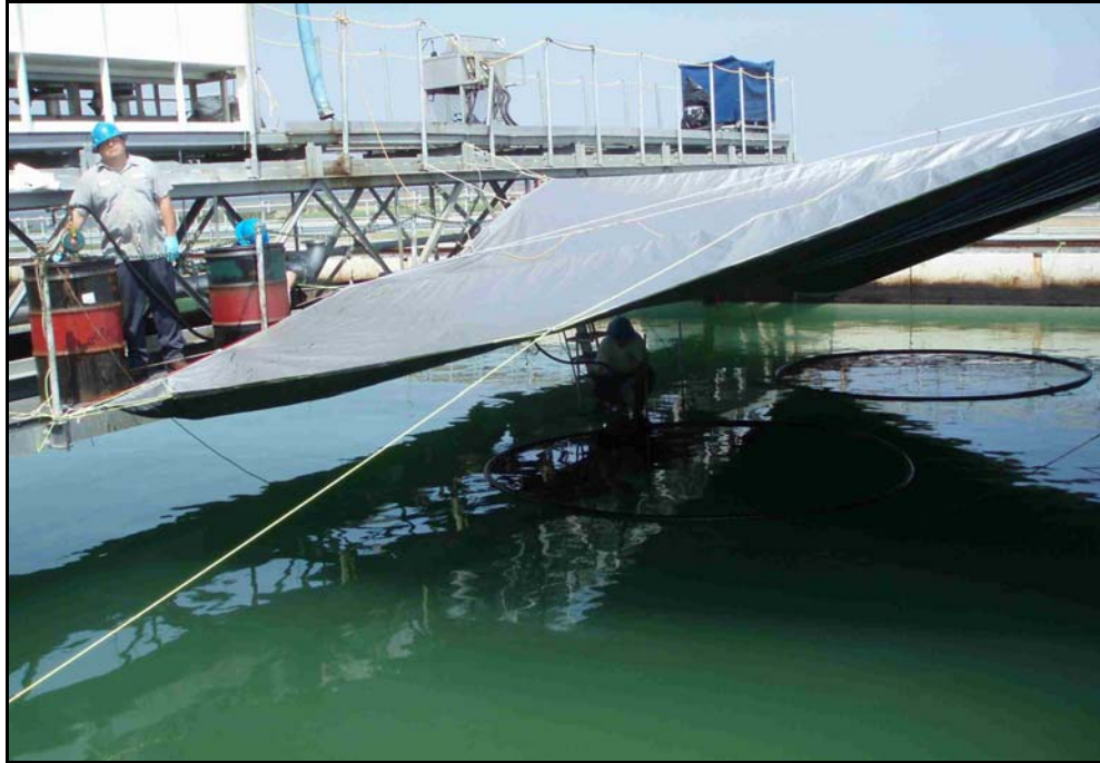
Figure 2. Photograph of the set-up for the work
