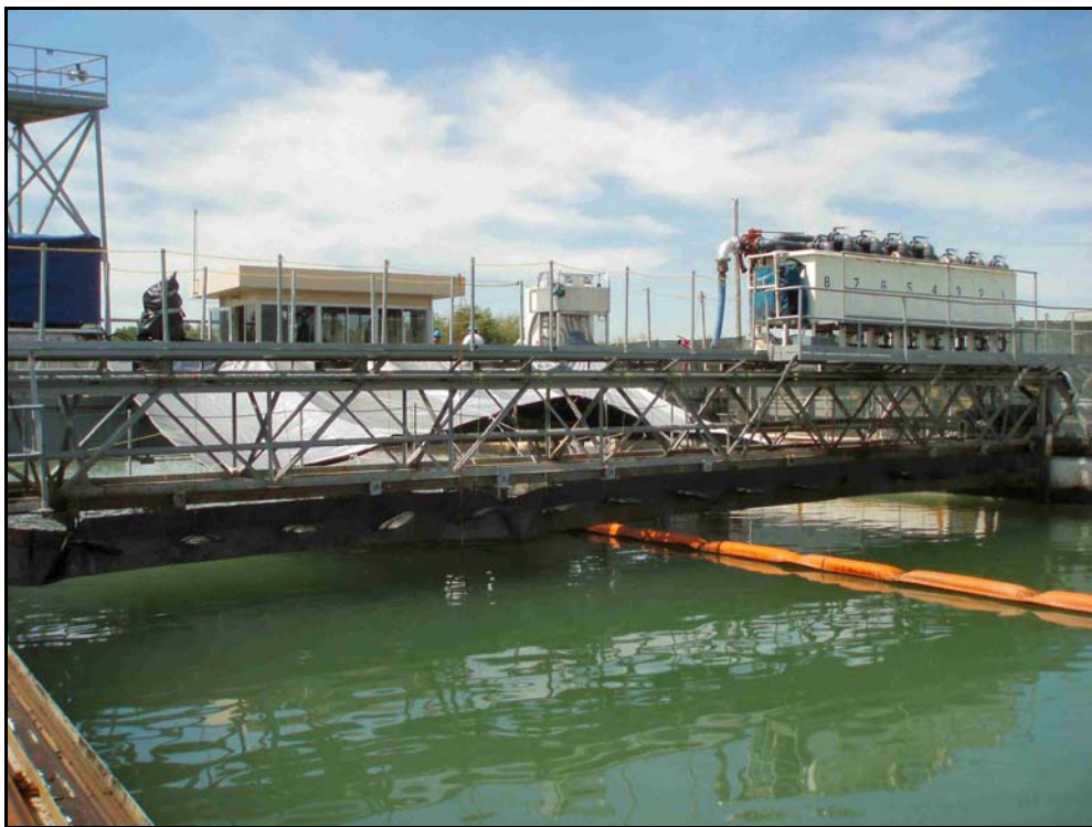
Figure 3. Boom was placed down the water surface
