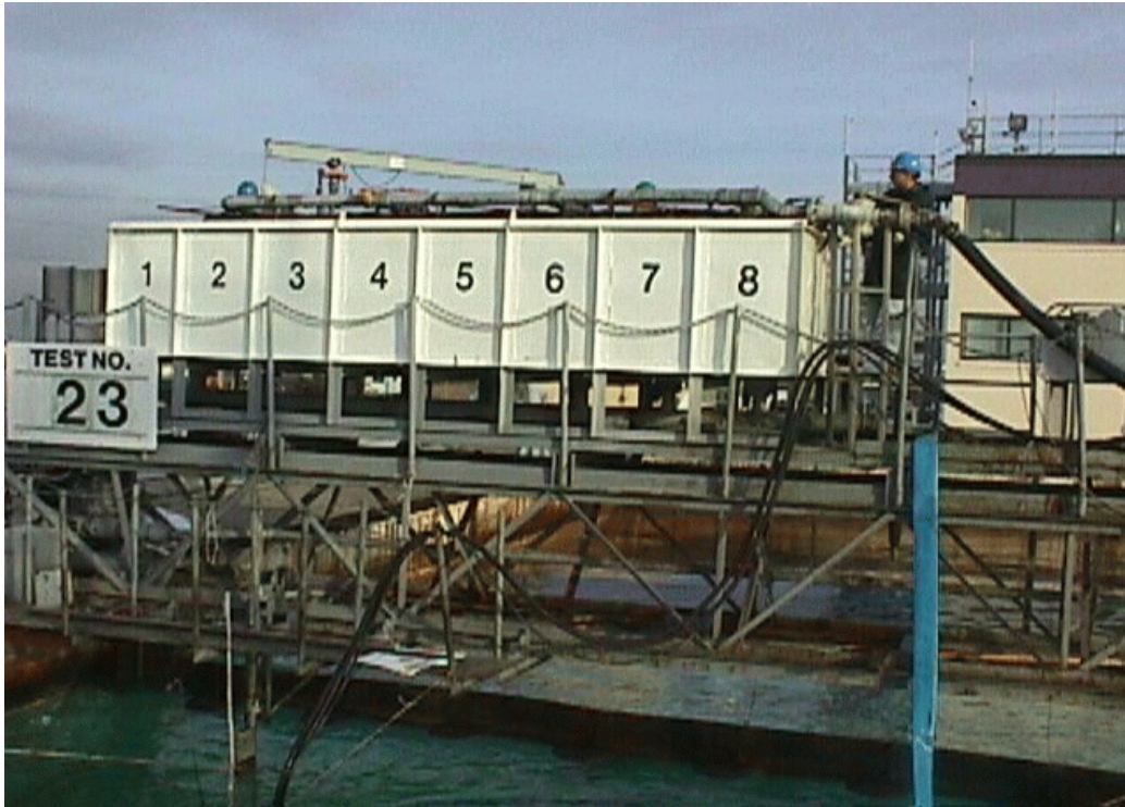
Figure 3. Recovery tank on auxiliary bridge.
