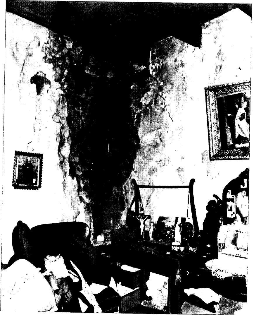
Leaky roofs are one of the major problems facing the limited-income elderly in New Mexico. Leaking roofs cause erosion of walls and the eventual collapse of the roof.
