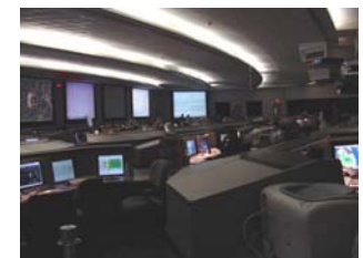
2 Operational Control Centers
