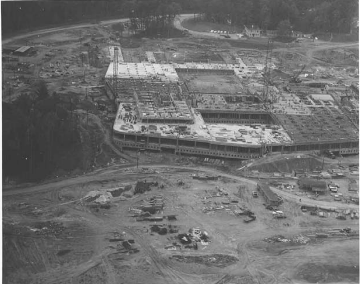
The state of construction in October 1959.
