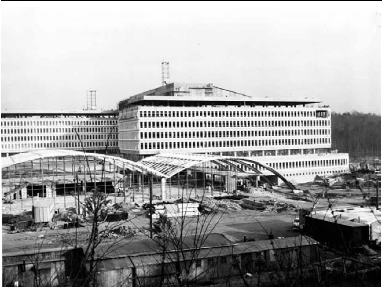
The cafeteria taking shape.
