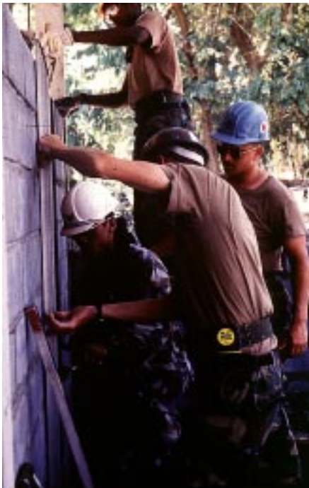
U.S. Army Pacific and Royal Thai Army engineers work side-by-side to construct a schoolroom during COBRA GOLD '97 in Thailand.
