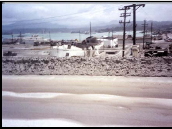
Buildings near the flight line at Cubi Point collapsed by the weight of the ash and mud from the Mount Pinatubo eruption, June 1991
