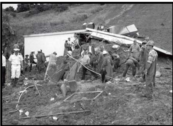
The collapsed roof and loading dock attest to the force of the mudslide which smashed into the station that morning. Here, an army of military and civilian personnel try to locate and recover the casualties.
