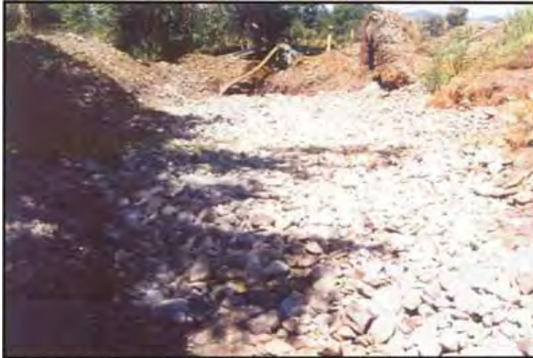
Figure 7. Cover over infiltration gallery (1998 Fields demonstration project for USBR).
