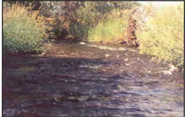
Figure 8. Infiltration gallery upon completion (1998 Fields demonstration project for USBR).
