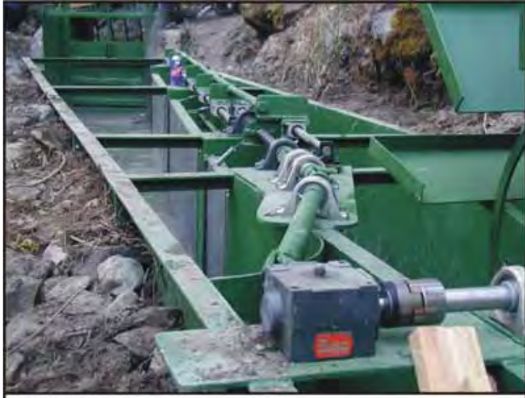
Figure 13c. Flat plate fish screen.
