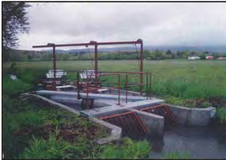
Figure 13a. Dual drum fish screen with trash rack.
