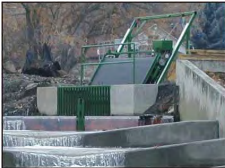
Figure 13d. Traveling belt fish screen.
