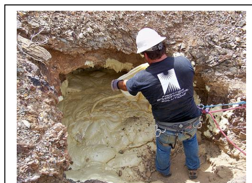
Photo 3. Installation of PUF in a shaft (photo taken by S. White 2009)
