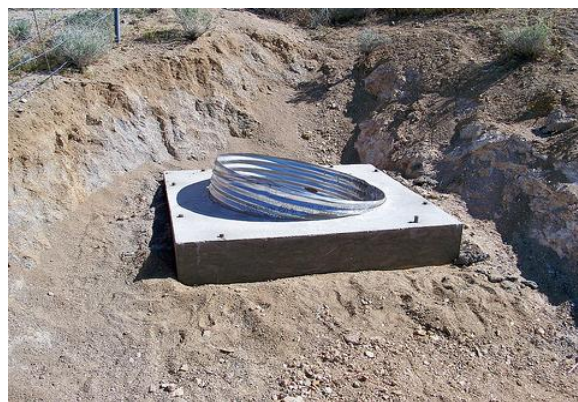
Photo 5. Culvert (36") recessed inside the portal of a shaft.
