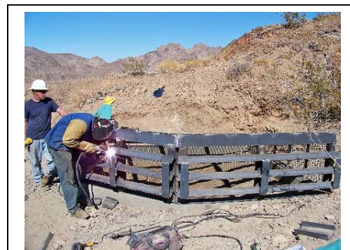
Photo 10. Installation of a cupola over the top of a shaft (photo taken by S. White,2009)
