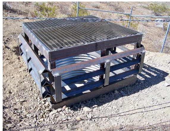
Photo 6. Cupola installed over the culvert (photos taken by S. White 2009)
