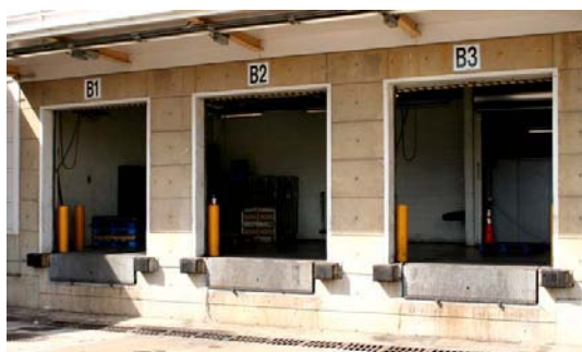
Appendix C Figure B-6—Loading Dock
