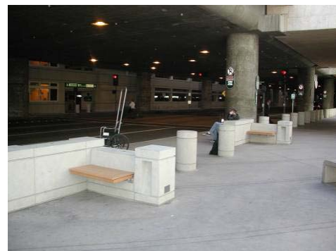
Appendix C Figure C-7 Vehicle Barrier—At Grade
