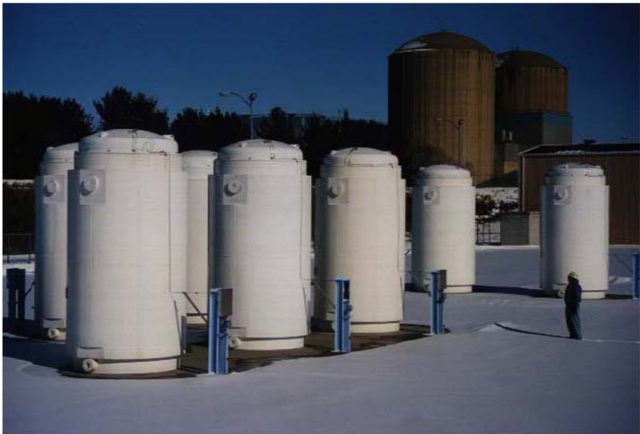
Figure 3-1 Series of Transnuclear (TN)-40 casks at an independent spent fuel storage installation.
