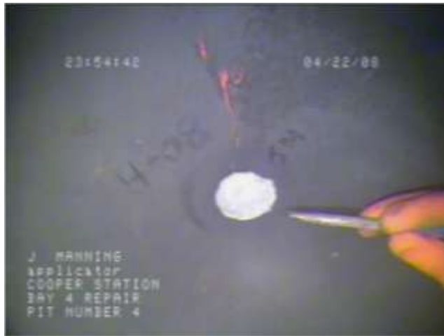
Figure C.1-2 Example of repair of pitting corrosion in torus
