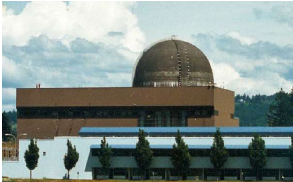
Figure 6-6 Trojan nuclear power plant posttensioned concrete containment
