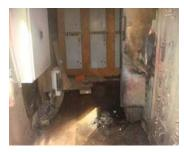
One miner was killed and two were seriously injured when they came into contact with a bottom feed circuit breaker as they were installing ground fault indicator lights in a circuit breaker enclosure.
