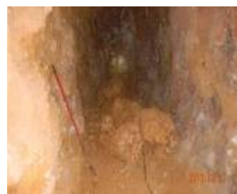
Victim was found approximately 250 feet inside the mine. He was working alone and had been struck by a fall of rib.
