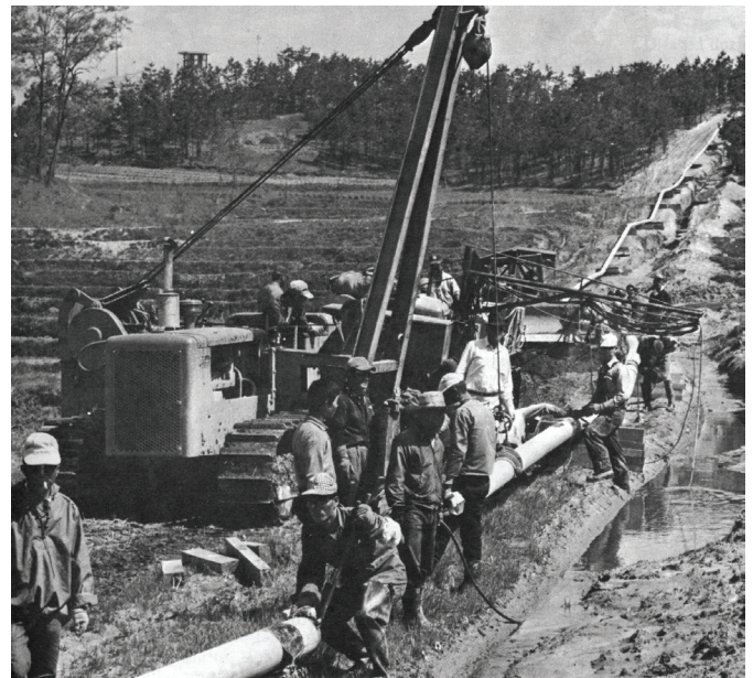
Laying out pipe for trans-Korea POL Pipeline, 1970
