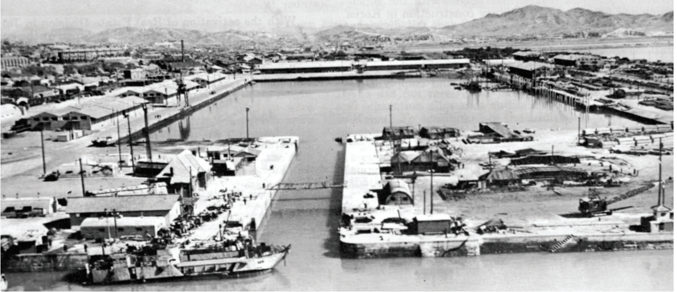
Tidal Basin Rehabilitation in Incheon, 1963. The mitre gates are undergoing repair on the south side of the lock. The piles used in the replacement of the south wharf can be seen in the right background.
