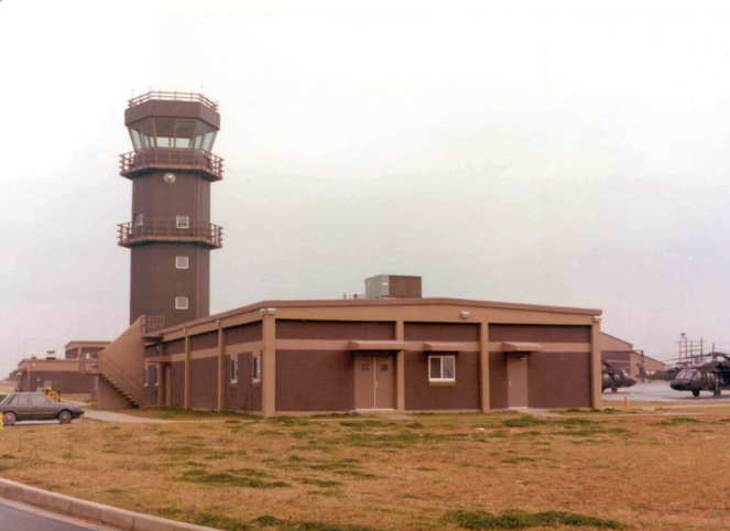
Operations Building, Camp Humphreys, 1984
