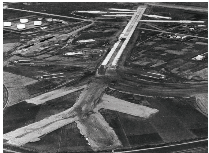
Partial completion of dispersal pads and associated paving, Kunsan, 1969
