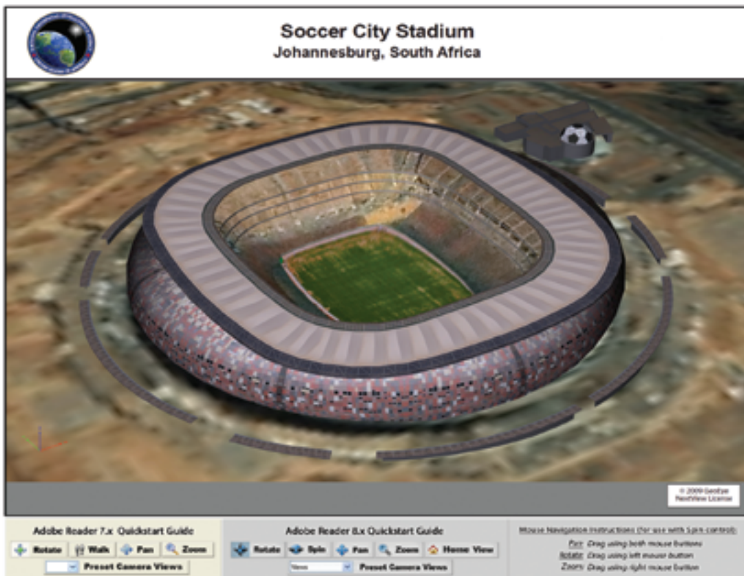
This image is a screen capture from NGA's 3-D scene visualization of the Soccer City stadium in Johannesburg, South Africa. The scene visualization is not static, it is an animation run from a database, giving the user the ability to zoom in and out, change the look angle and fly or drive around the structure.
