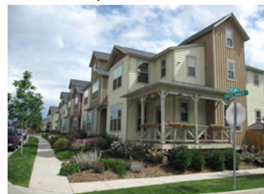
Edwards, Colorado, courtesy of Clark Anderson
