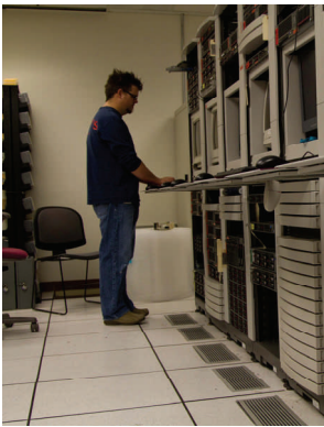
Preparing for the move
