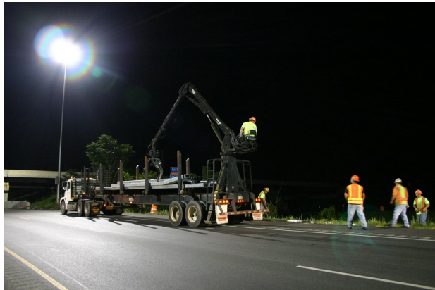
Figure A-2.2. Crew working on the installation of guard rails. It can be appreciated in the photographs the high light levels and uniformity provided by the lighting. [Photo credits: Dennis Guyon, Lighting Research Center]
