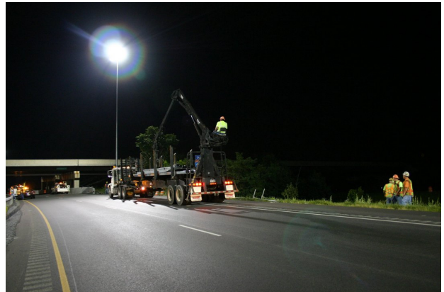
Figure A-2.2. Crew working on the installation of guard rails. It can be appreciated in the photographs the high light levels and uniformity provided by the lighting. [Photo credits: Dennis Guyon, Lighting Research Center]
