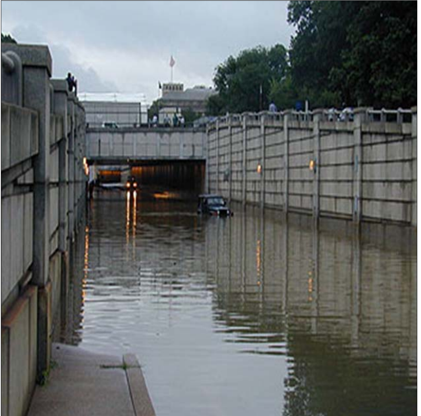
Effects of flooding on 9th Street, NW in downtown Washington, DC in June 2006.
