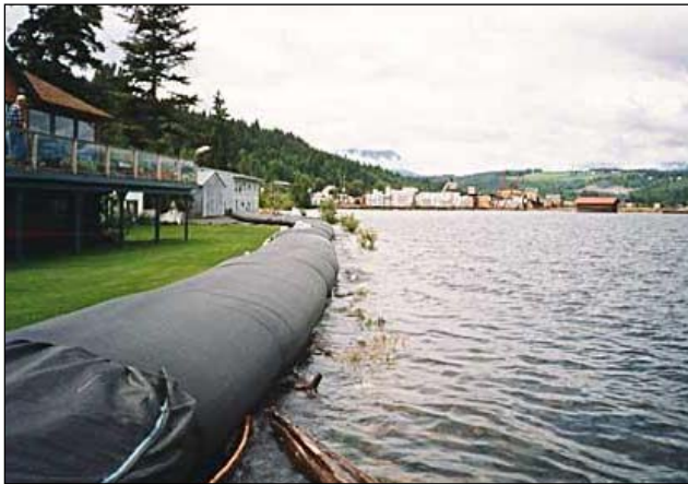
The pictures above depict temporary dams, an inflatable dam (left) and a port-a-dam (right).
