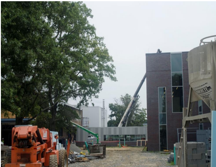
Test Lab Renovation Project
