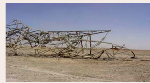
Damaged transmission tower, 2003
