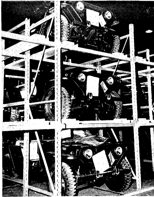
Figure 5-18 Roll-through racks for stacking vehicles in storage
