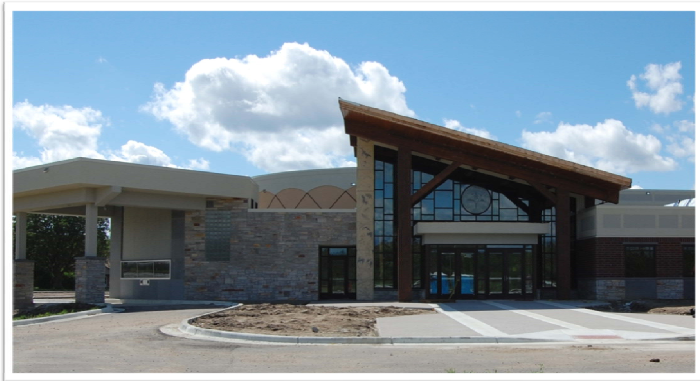
Bois Forte Community Facility — Construction progress August 2010
