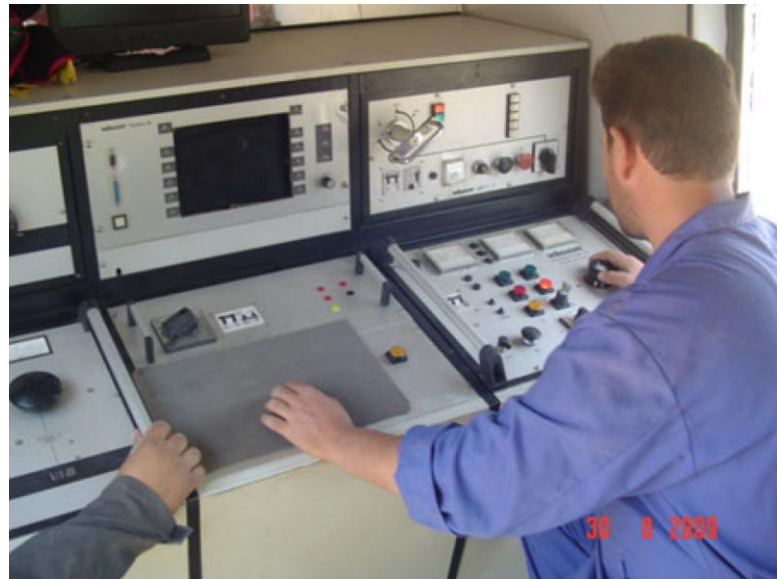
Site Photo 5. Contractor-provided training of MOE operators (Courtesy of GRC)
