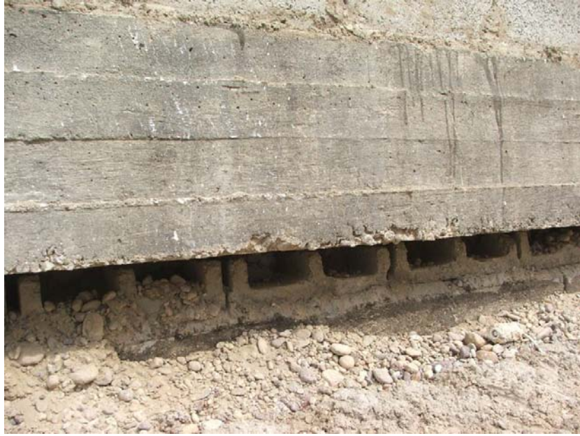
Site Photo 5. Course of CMUs placed with cores horizontal
