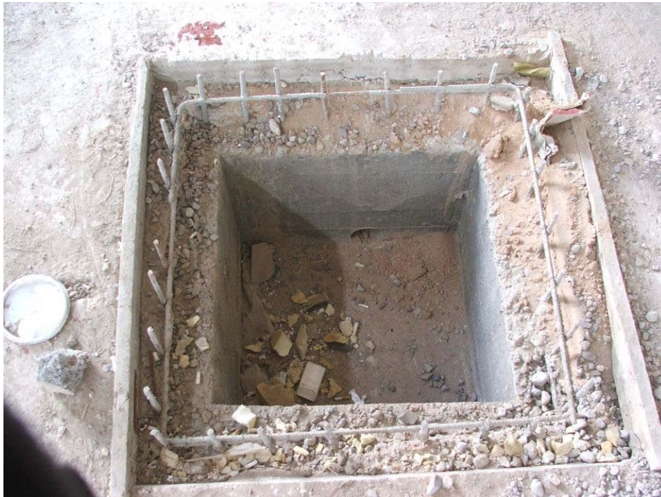
Site Photo 12. Cast-in-place sanitary sewer manhole
