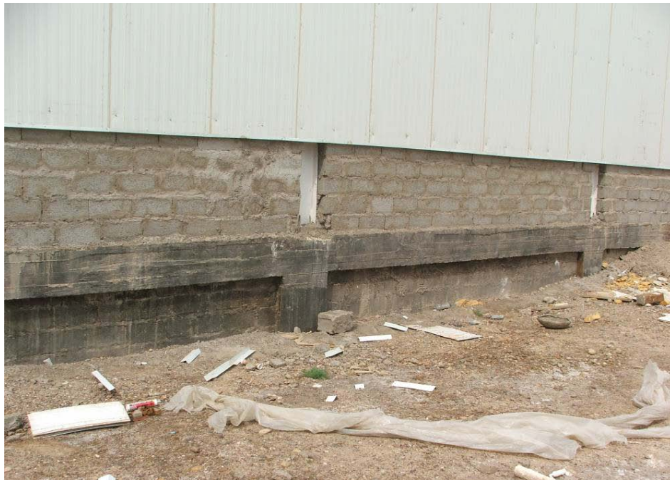
Site Photo 3. Perimeter CMU wall
