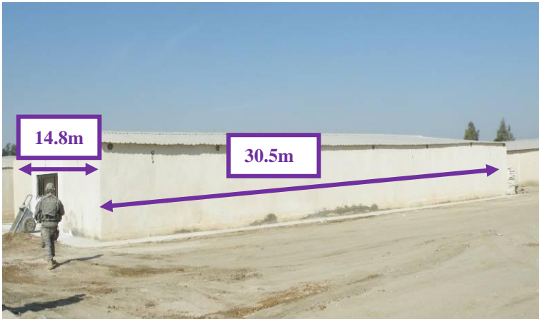
Site Photo 7. Exterior view of the training facility
