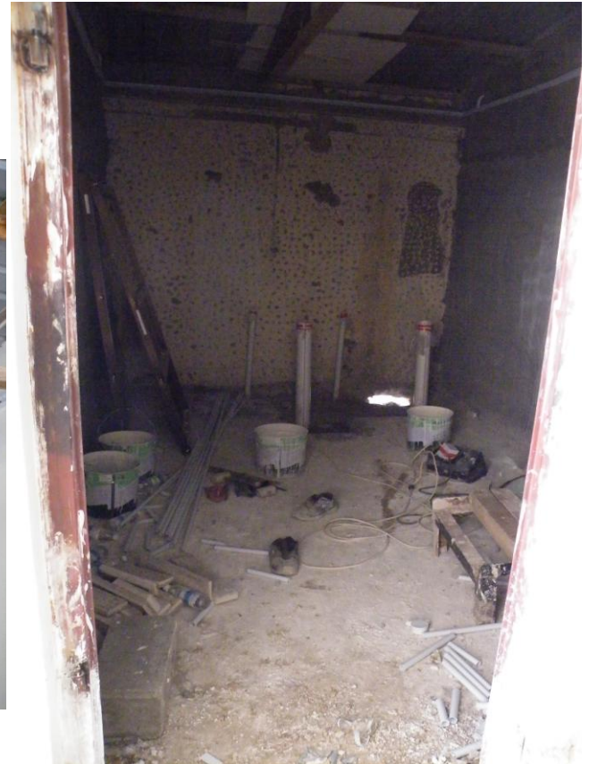
Site Photo 10. Current condition of bathroom
