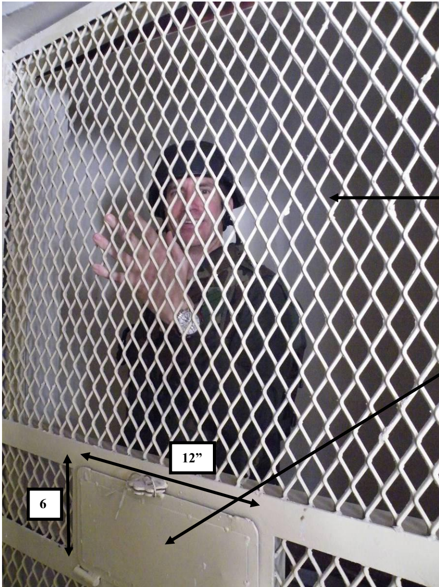
Site Photo 6. SIGIR Inspector testing quality of cell door
