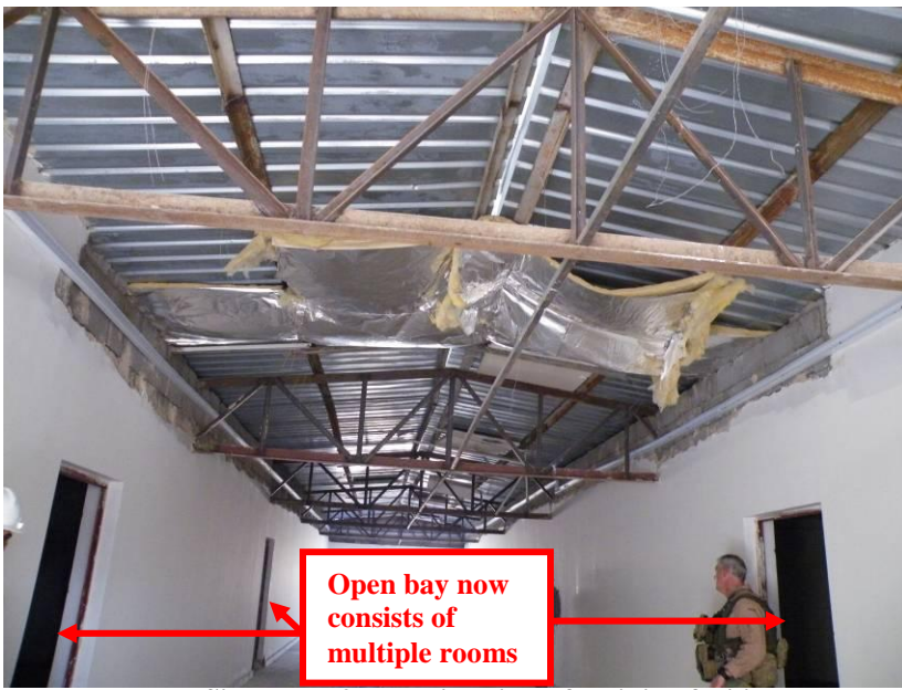
Site Photo 9. Interior view of training facility
