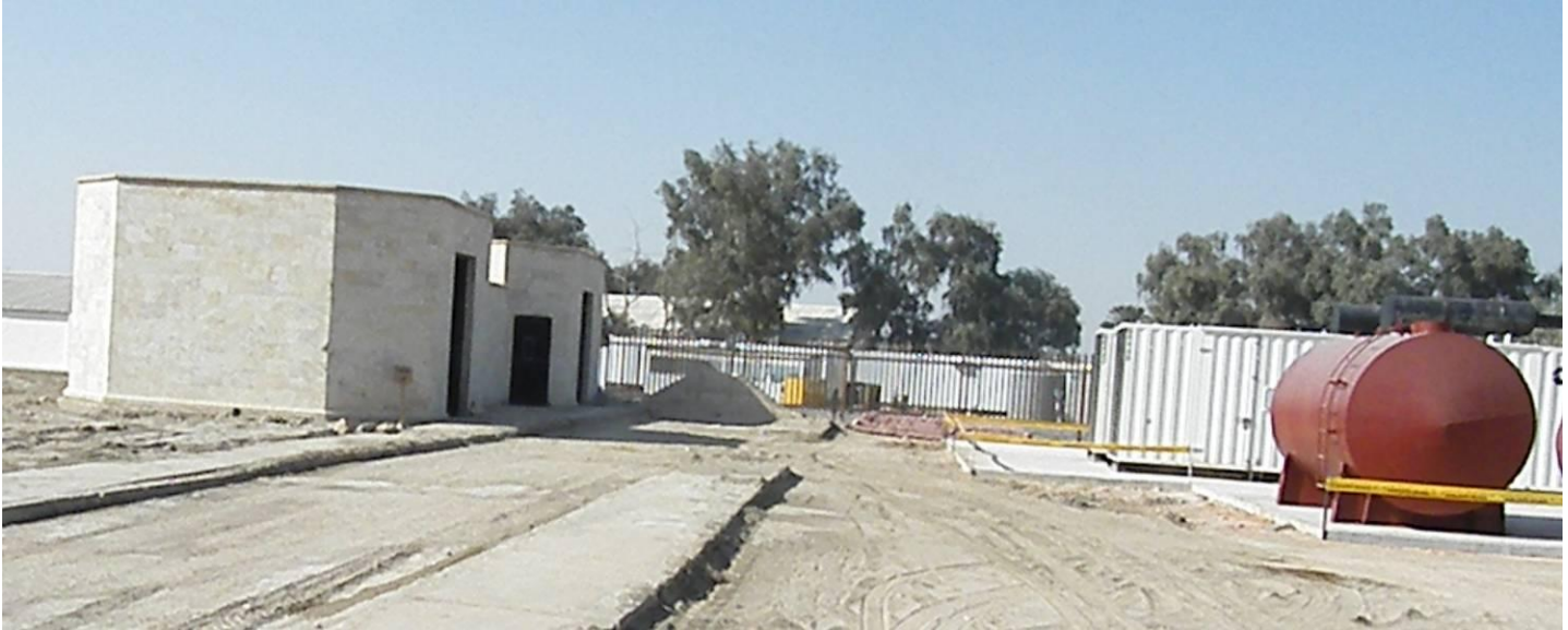
Site Photo 11. Exterior view of the generator facility
